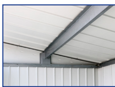
Strong Steel Roof Truss
